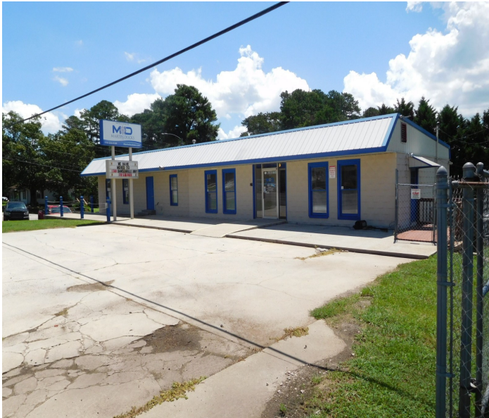
Browns Bridge road frontage
